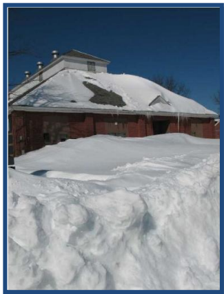
Waterbury State Offices, March 8 th , 2011
